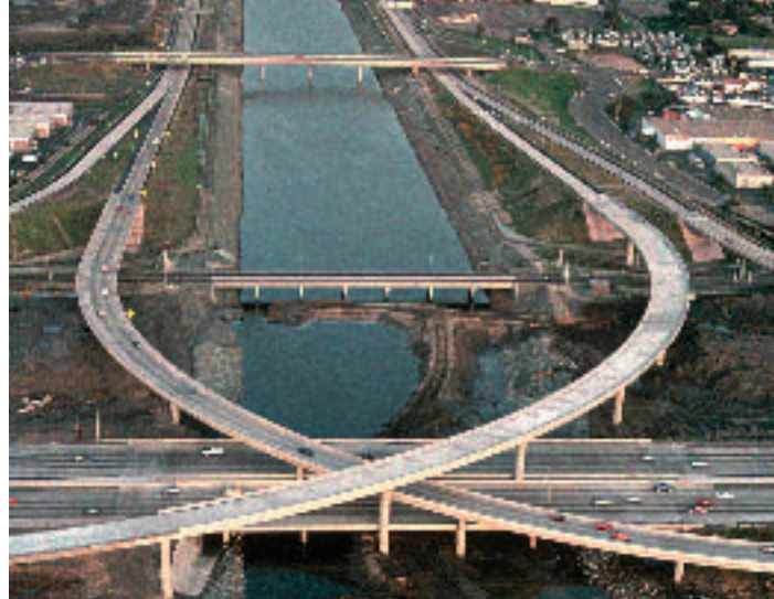
Figure 10 Channelizing a stream involves removing Earth materials to straighten and deepen the stream channel.
