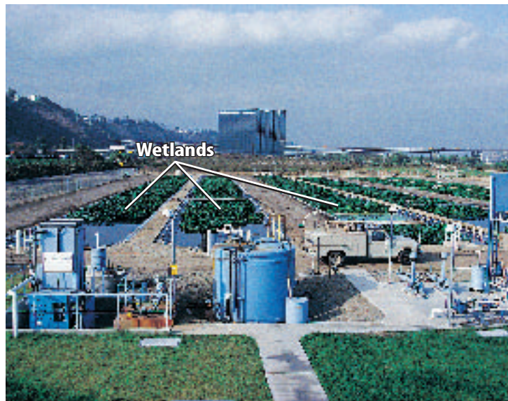
Figure 18 Wetlands at this sewage-treatment facility are used to remove nutrients before water flows back into the environment.
