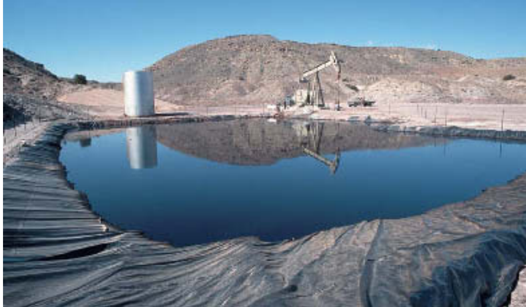
Figure 13 Properly lined holding ponds reduce the chances of groundwater pollution.
